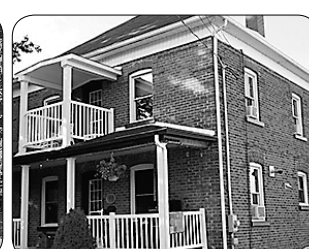
47, 1RE AVENUE, WINDSOR COTTAGE 4CC, BCP DE BOISERIES.
